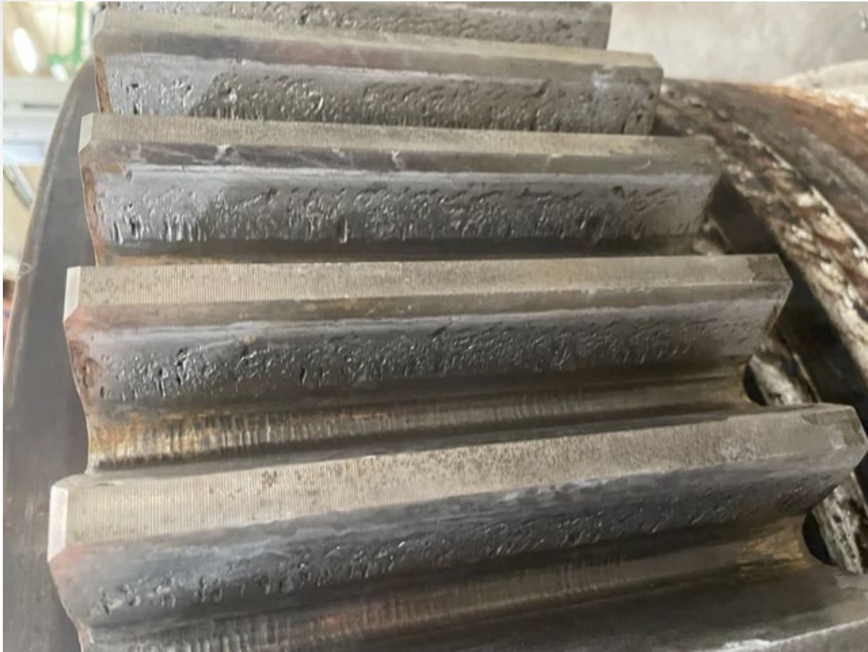
Pitted north drum gear
